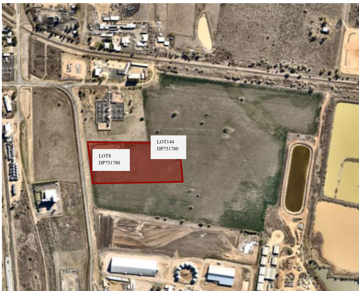
Figure 1 - Existing Site Context
